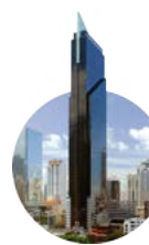
2012 Tower Financial Center
