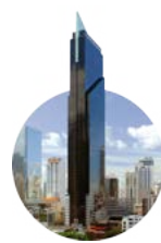
2012 Tower Financial Center
