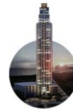
The Regent Under construction.
