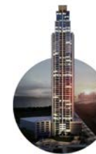
The Regent Under construction.
