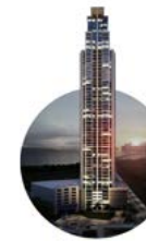
The Regent Under construction.
