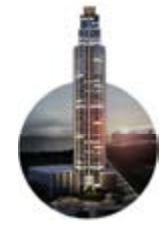
The Regent Under construction.
