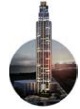
The Regent Under construction.
