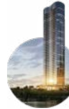
Skyline Under construction
