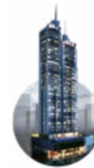
The Tower Under construction
