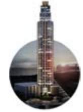
The Regent Under construction.
