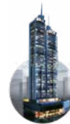
The Tower Under construction
