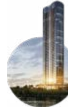
Skyline Under construction
