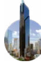
2012 Tower Financial Center
