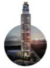
The Regent Under construction.
